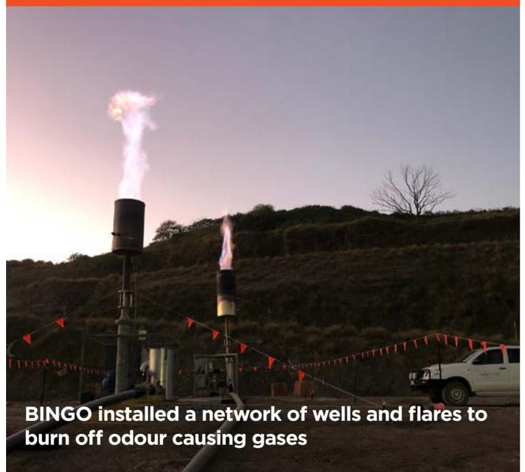
**BINGO installed a network of wells and flares to burn off odour causing gases**
